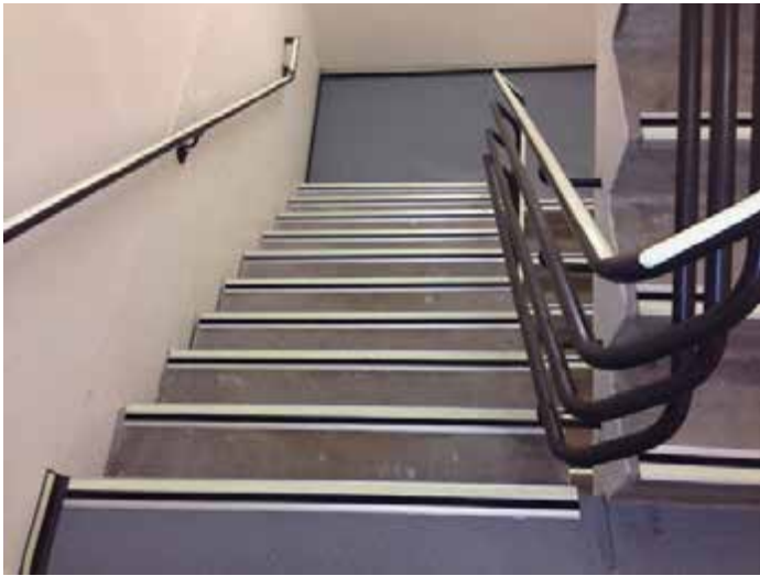
UL1994-listed photoluminescent egress path markings since 2009. (Photo: Copyright PERMALIGHT®.)
