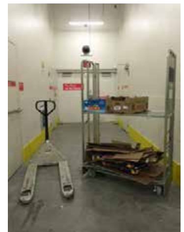
Figure 1: Blocked means of Egress (Photo courtesy of Scott Tobias.)
