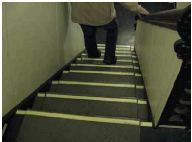
NYC high-rise office building exit path markings 2005. (Photo: Copyright PERMALIGHT®.)
