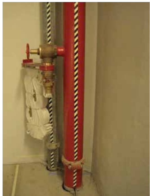
Photoluminescent Obstacle Marking 2014. (Photos: Copyright PERMALIGHT®.)
