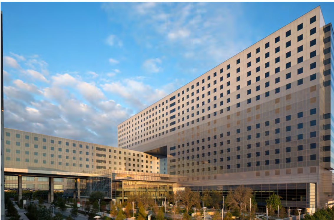
The new Parkland Hospital encompasses a 2.8 million square foot campus and includes an 862-bed hospital, outpatient center, parking garage, central utility plant and logistics building. Architect: Hdr + Corgan © : 2014 Assassi Production
