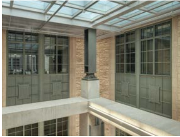
A fire-rated glass floor system transfers light into Northwestern University's Engineering Life Sciences infill. Technical Glass Products Photo
