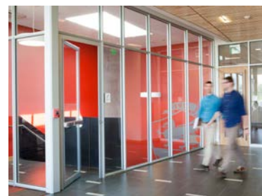
Fire-rated glazing systems have the unique ability to limit the spread of fire in expansive buildings while maintaining an open feel.
