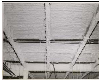
A Great Finished Deck
