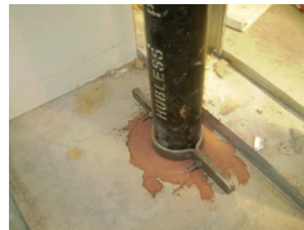
Finished installation, with piping clamps. Hamilton-Benchmark Photo
