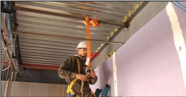
Safety is important for firestop - containment workers. FCIA Photo
