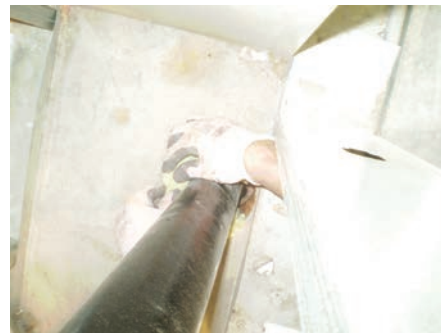
Installing mineral wool 'packing/forming' material. Hamilton-Benchmark Photo
