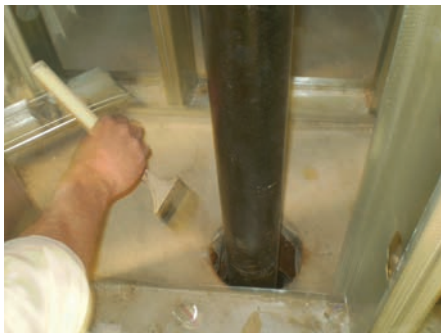
Cleaning the area to receive the firestop products. Hamilton-Benchmark Photo
