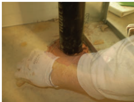
Installed firestop sealant is 'tooled or smoothed' per manufacturers published installation instructions. Hamilton-Benchmark Photo
