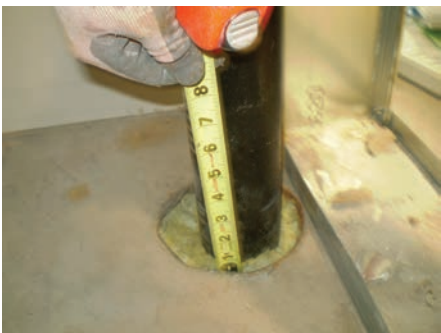
Measuring the depth left for firestop sealant. Hamilton-Benchmark Photo
