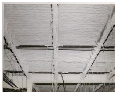
A Great Finished Deck
