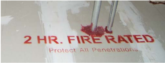
Painted stencils can mark walls and comply with code. Multicon photo
