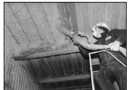
Applying the Proper Thickness
