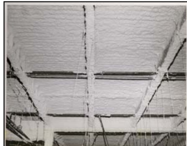
A Great Finished Deck
