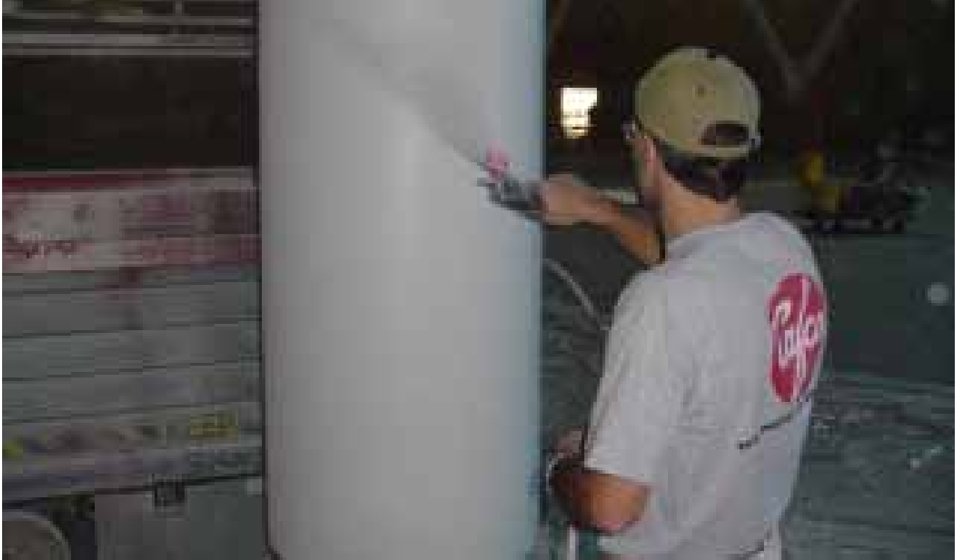
Intumescent coating being applied to large tube steel columns. ISOLATEK photo
