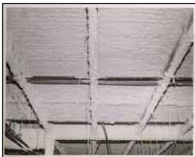
A Great Finished Deck
