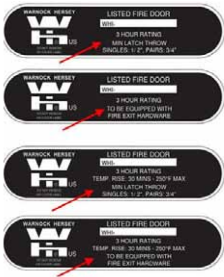
Examine labels on door and frame. DHI Photo
