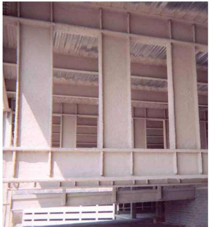
Medium Density, wet spray SFRM applied to structural members. ISOLATEK photo
