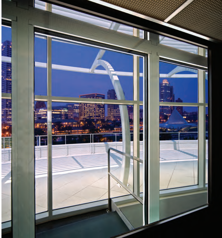
Fire-rated glazing can separate spaces, as allowed by code. - TGP Photo
