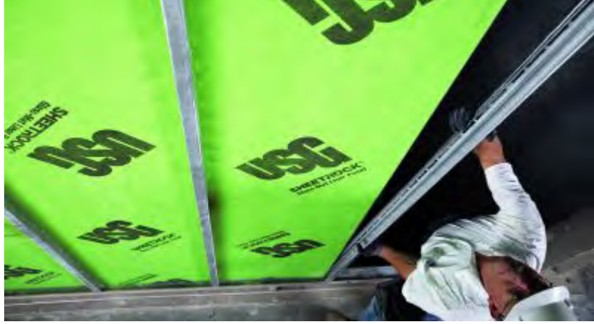
Stud spacing, fastening patterns and gypsum board type and thickness is important to complete a fire-resistance rated wall assembly. - USG Photo
