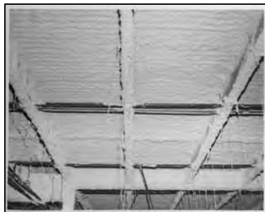
A Great Finished Deck
