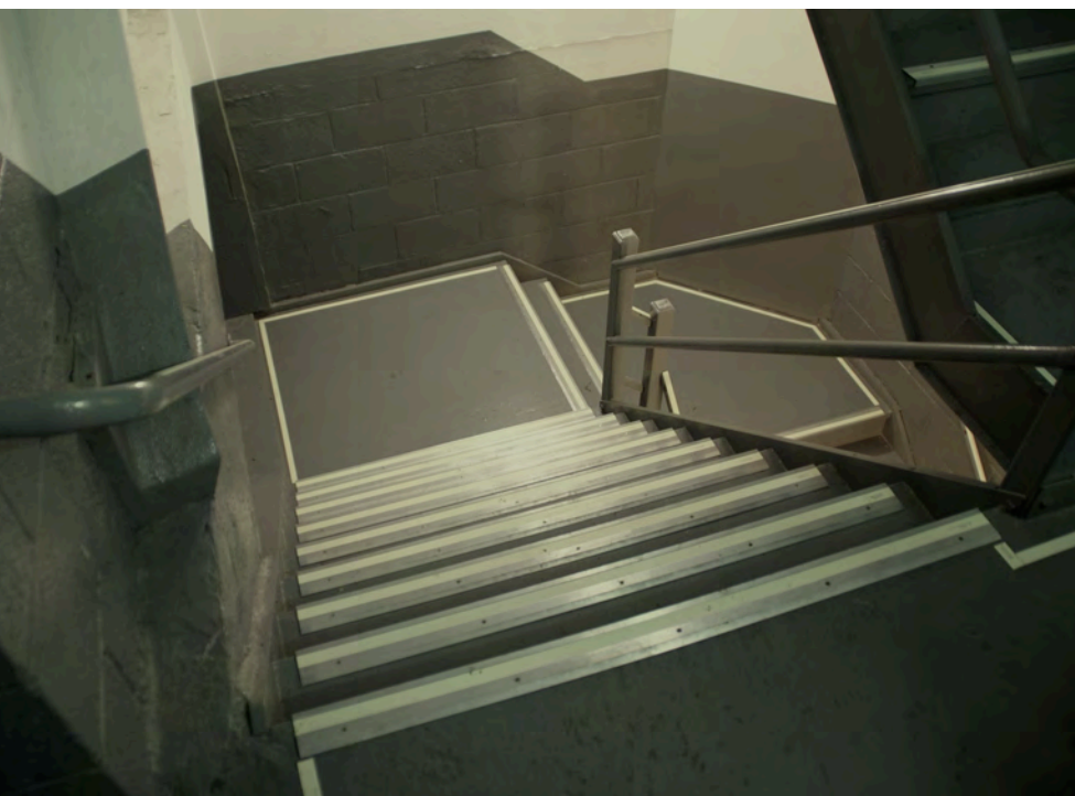
Stairwell under lighted conditions.
