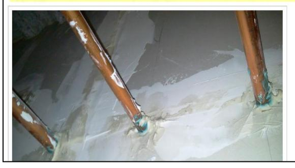
ASHE is urging facility managers around the country to check their copper pipes for signs of corrosion. If you have experienced a sealant that corroded copper medical gas or water pipes, or if you have any other insights to offer about this issue, please contact ASHE at advocacyhighway@aha.org. Feel free to pass this information to
