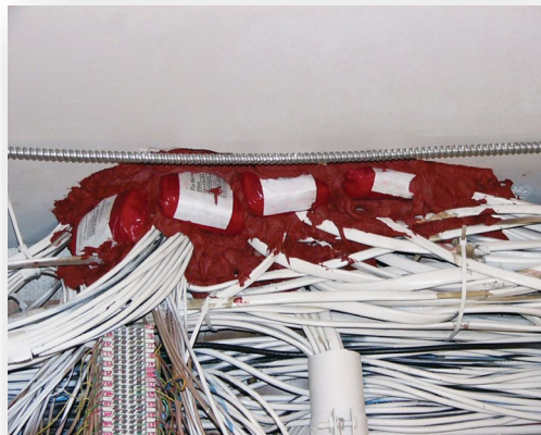
Multiple products / Excessive cable load
