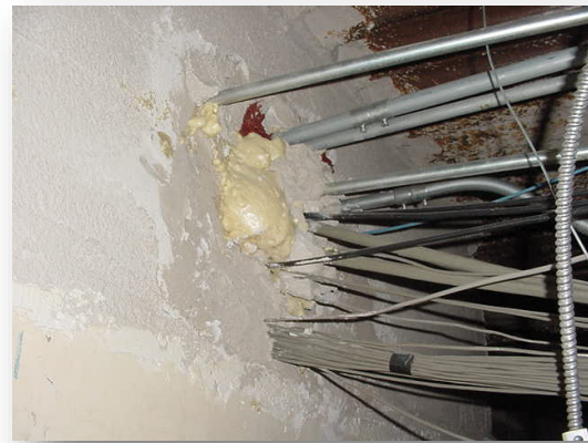
Resealed with combustible foam, not firestop
