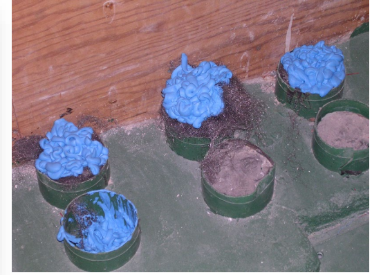
Inadequate dose, and un-tooled material
