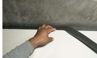
Foam Strips are an Intumescent with Foam expansion and compression capabilities for joints requiring up to 100% movement.
