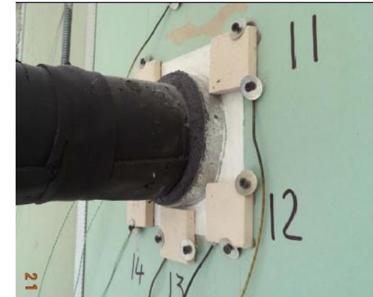
e 3 – Intumescent sealant between the insulation and GS sleeve has started to
