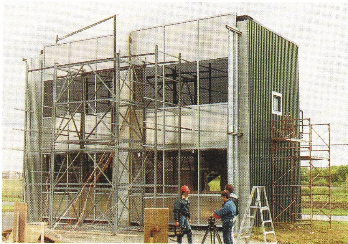
Fig. 1. Face of full-scale, permanent, fire-test facility at USG Corporation Research Center is set up for curtain wall fire test. Metal frame supports thermocouples for measuring flame plume temperature. Left side is “THERMAFIBER Curtain Wall Insulation Unit”; right side is “Glass Fiber Unit.”
