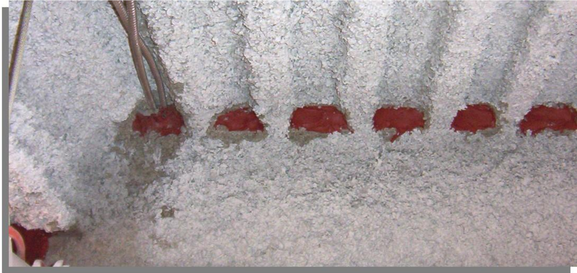
Firestop Solutions Photo
