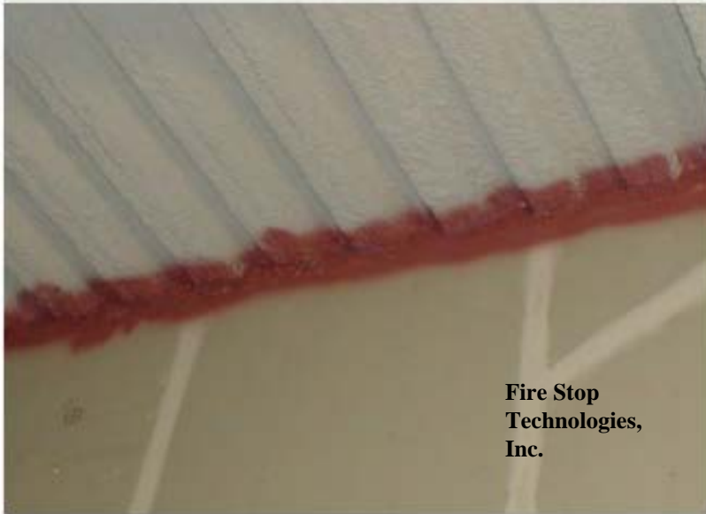
Fire Stop Technologies, Inc.
