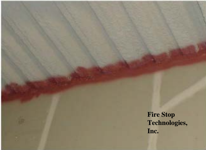
Fire Stop Technologies, Inc.
