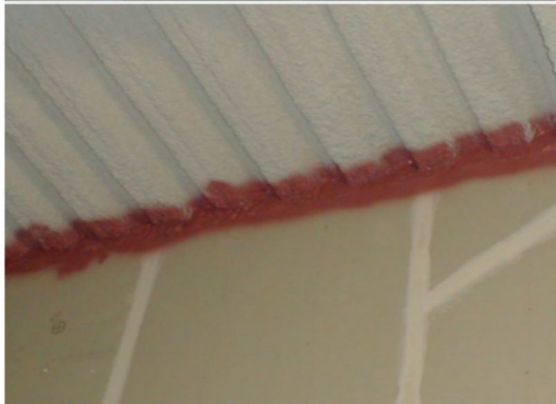
Fire Stop Technologies, Inc.
