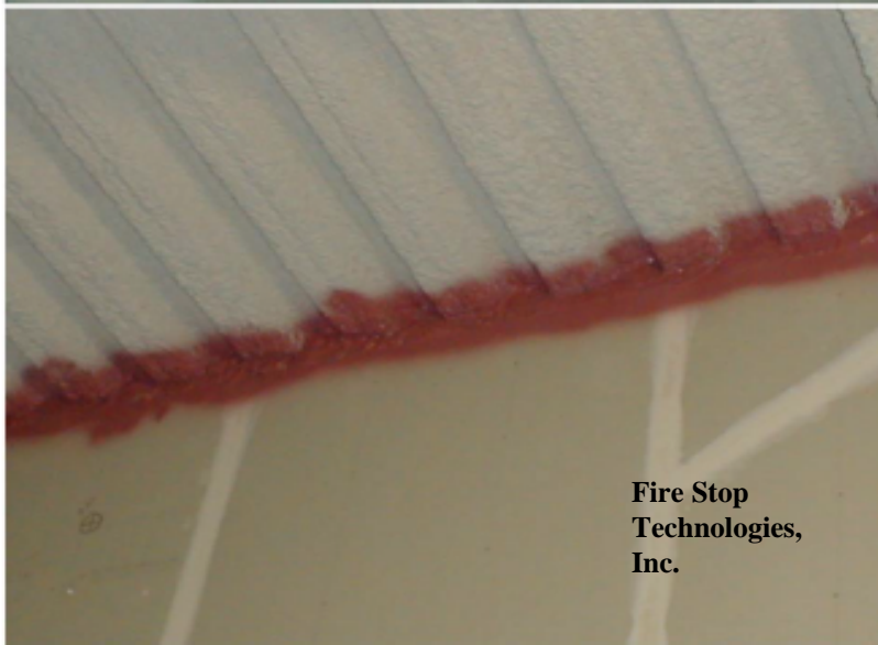
Fire Stop Technologies, Inc.
