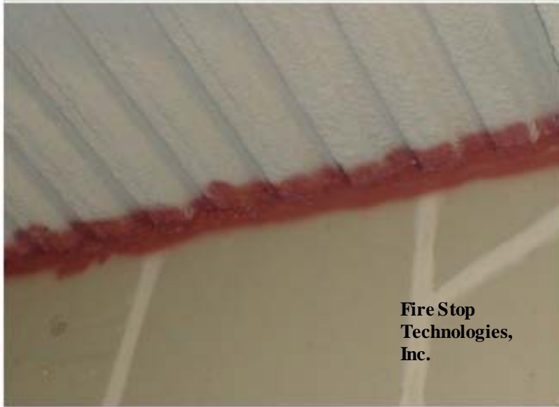
Fire Stop Technologies, Inc.
