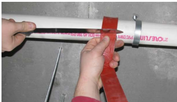
Wrap Strip is cut and ends 'budded'.
