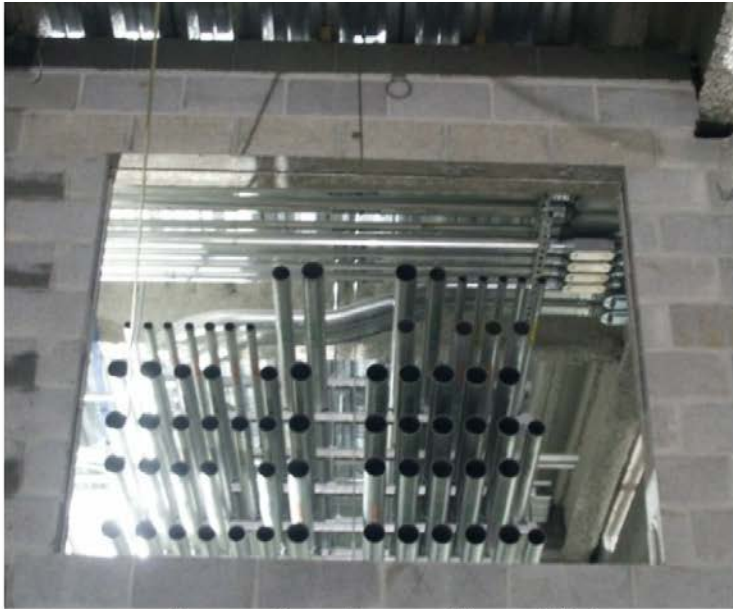
Large Openings with multiple penetrating items. PPMI Photo
