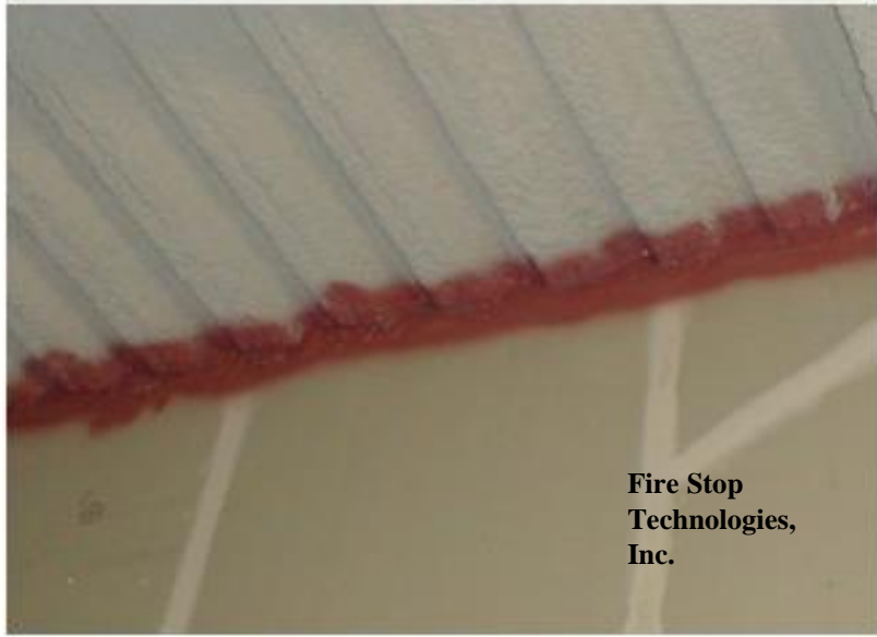
Fire Stop Technologies, Inc.
