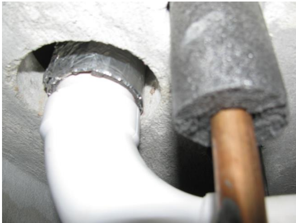
Annular space measurement and wrap strip application is critical.
