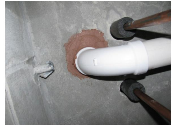
Firestop Sealant is applied, then tooled/smoothed for wetting into the surfaces to finish the firestop. Hamilton Benchmark Photos
