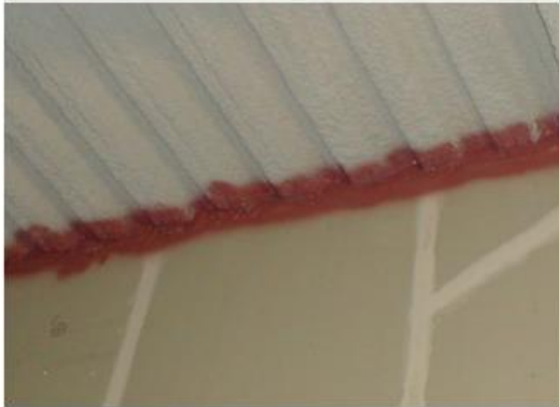
Fire Stop Technologies, Inc.
