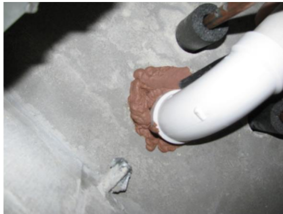
Firestop Sealant is applied, then tooled/smoothed for wetting into the surfaces to finish the firestop. Hamilton Benchmark Photos
