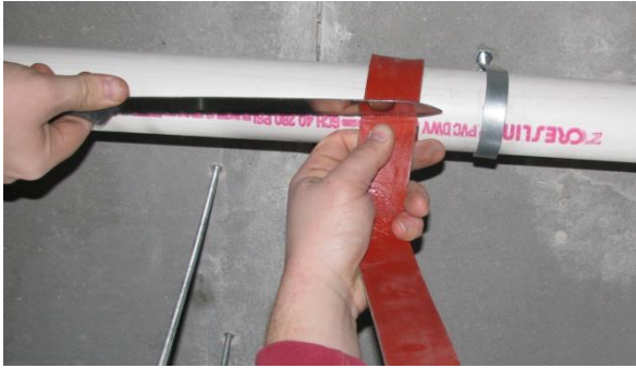
Wrap Strip is cut and ends 'buted'.
