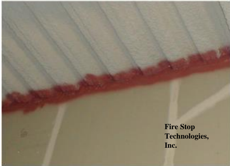
Fire Stop Technologies, Inc.
