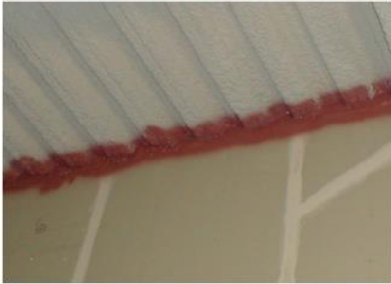
Fire Stop Technologies, Inc.
