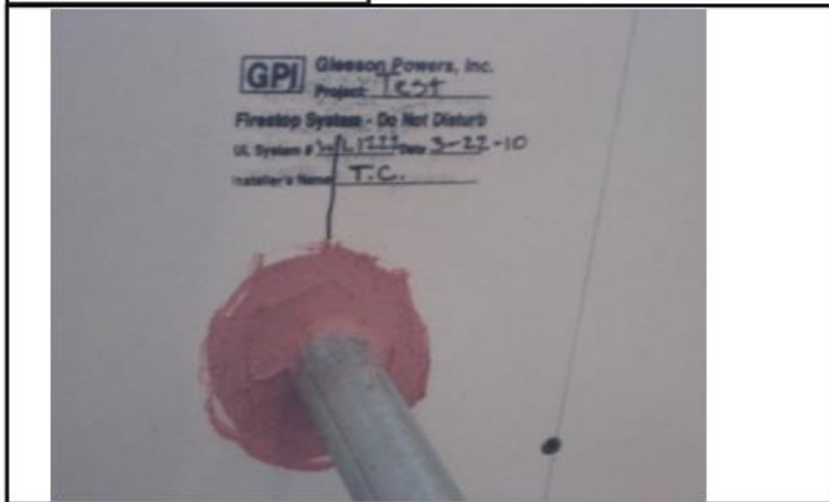
Corrective Action Photo
