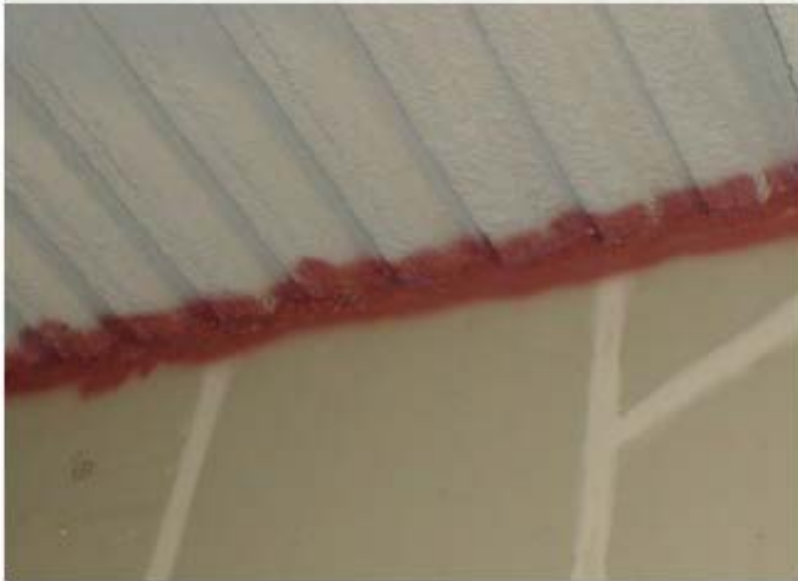
Fire Stop Technologies, Inc.
