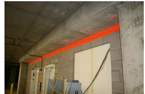
Firestop Southwest Photo
