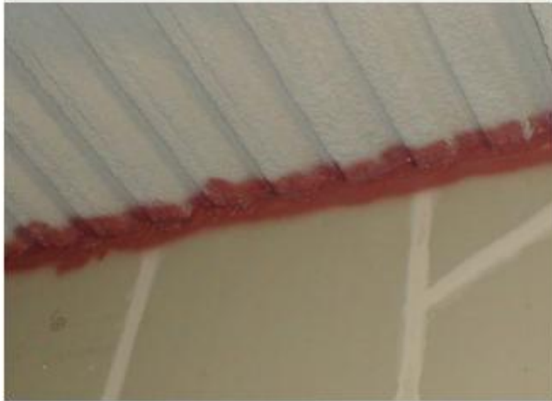
Fire Stop Technologies, Inc.
