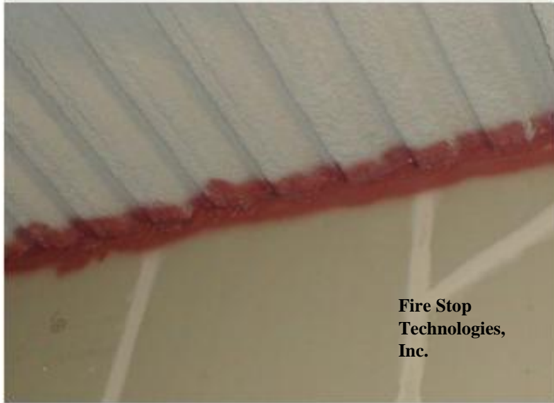
Fire Stop Technologies, Inc.
