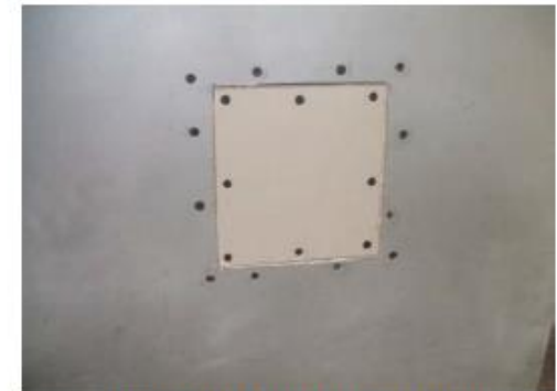
Figure 4: Apply Gypsum Panel Patch
