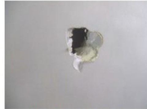
Figure 1: Damaged Gypsum Panel
