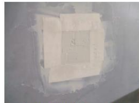
Figure 5: Tape and Finish Patched Area
