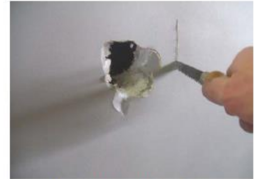
Figure 2: Square Off Damaged Area
