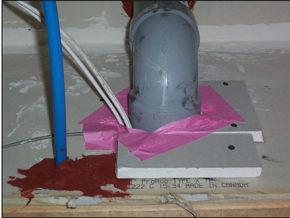
Affinity Firestop Photo Patches & Tape? Really?
