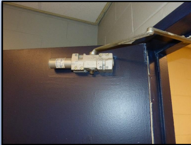
Missing Cover on Door Closer
