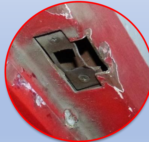
Damaged Strike Plate for Self-Latching Flush Bolt
