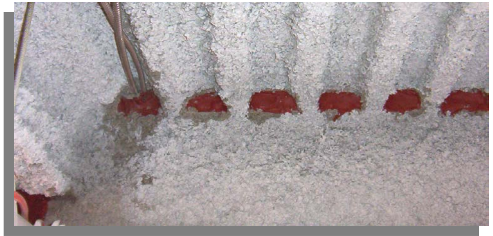
Firestop Solutions Photo
