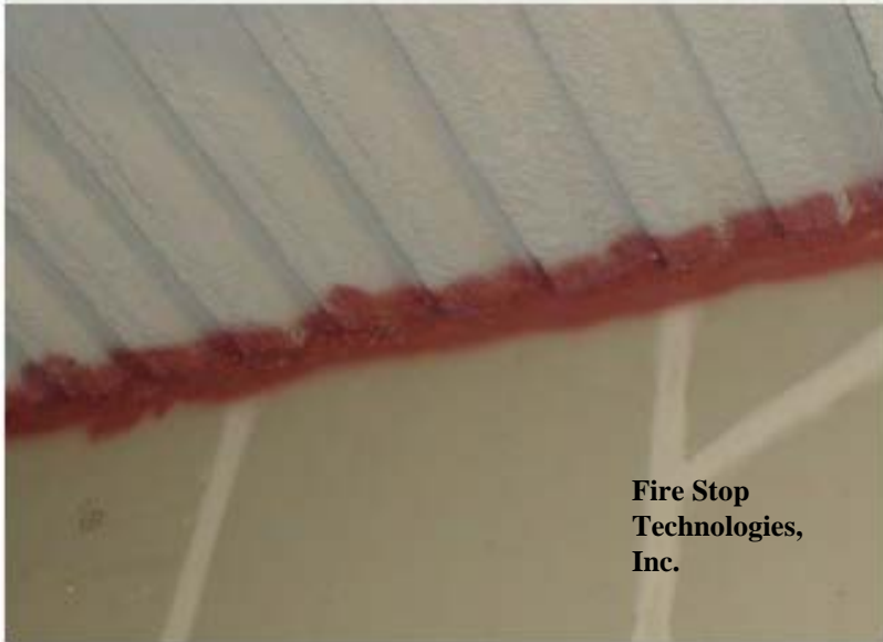
Fire Stop Technologies, Inc.
