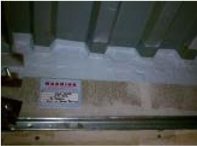
Performance Firestop Photo
