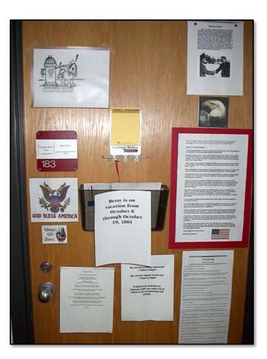
Fasteners penetrate door skin and product adds fuel to fire door assembly.
