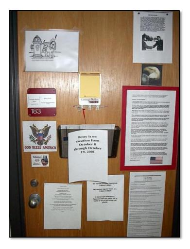
Fasteners penetrate door skin and product adds fuel to fire door assembly.
