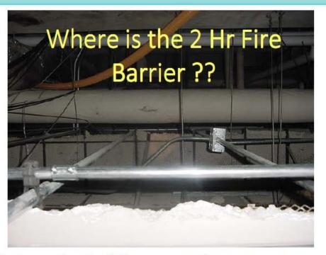
The Wall above the building separation was not constructed from floor slab to ceiling deck, therefore, non compliant
