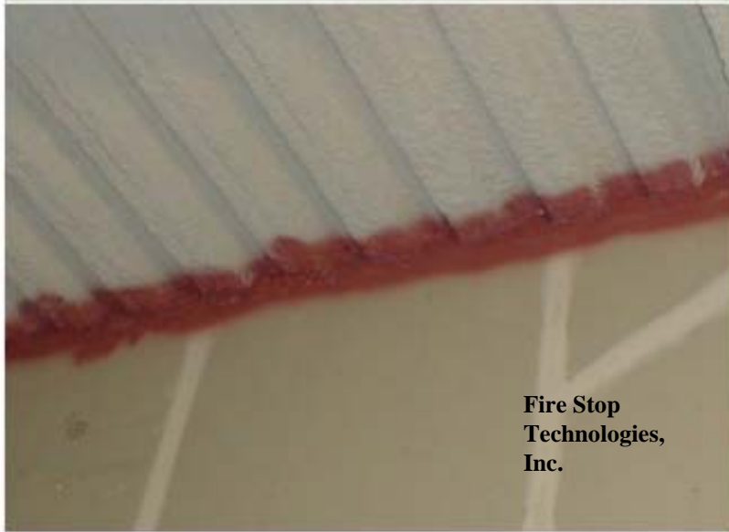
Fire Stop Technologies, Inc.
