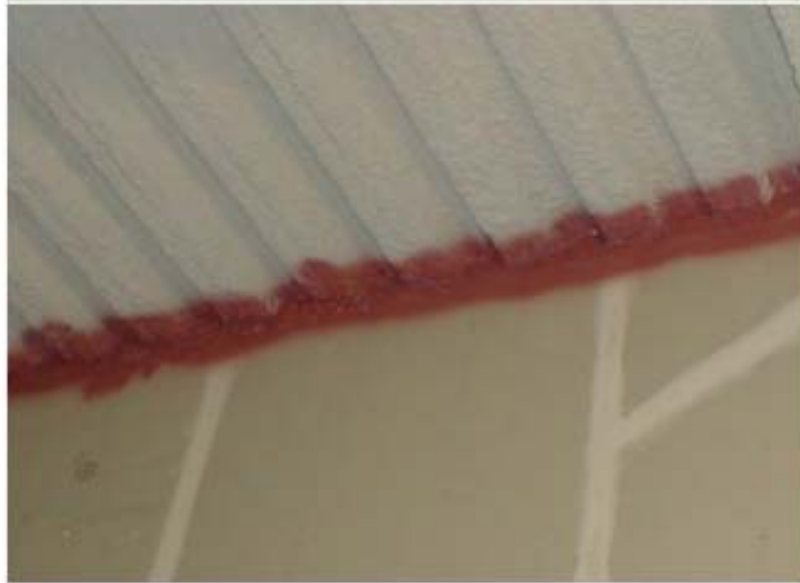
Fire Stop Technologies, Inc.
