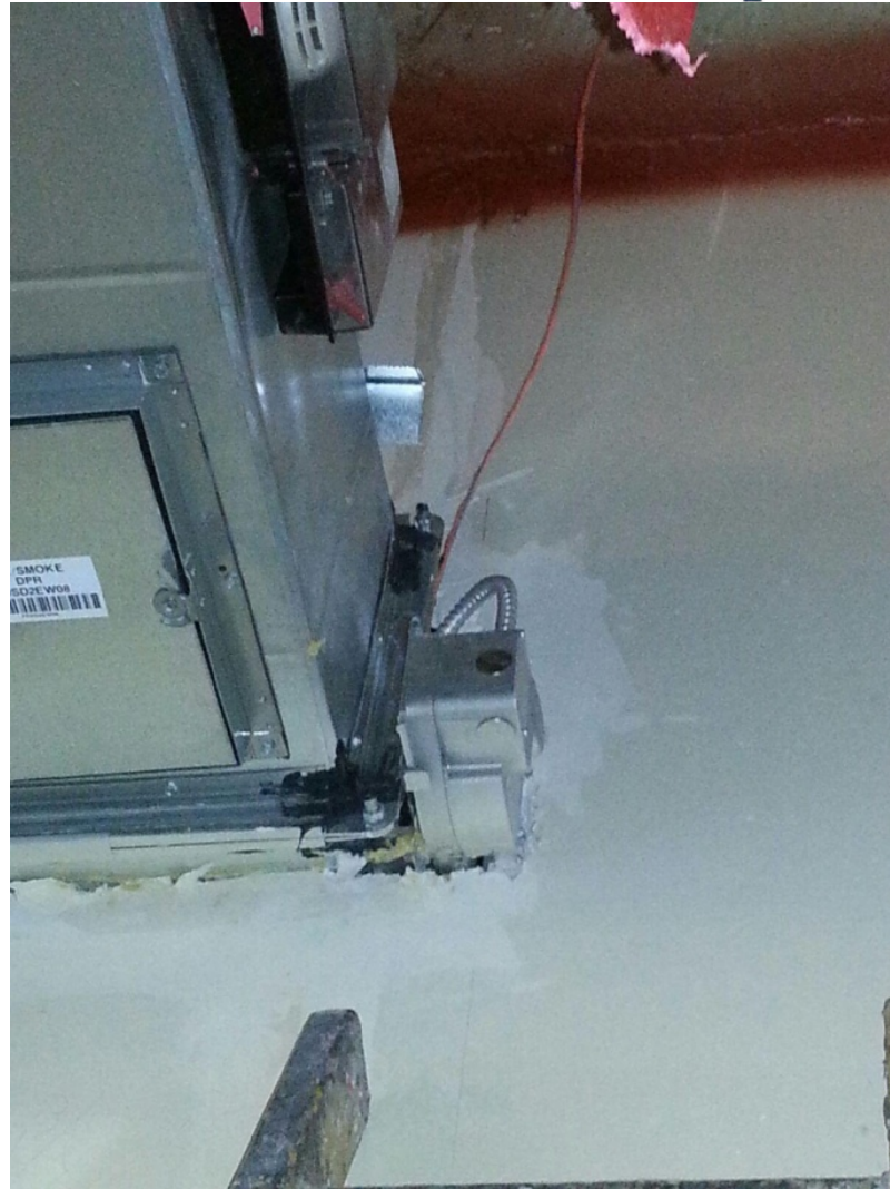
Actuator in the barrier.
