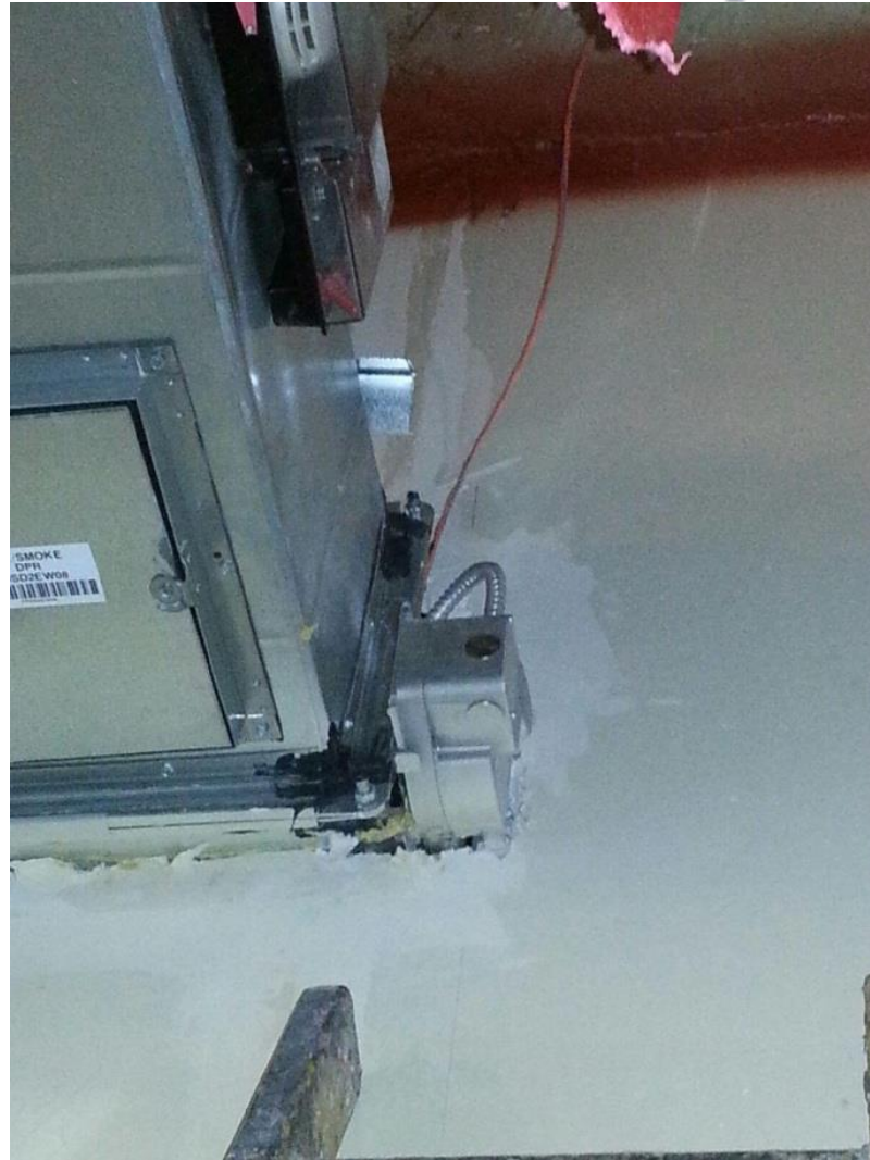
Actuator in the barrier.
