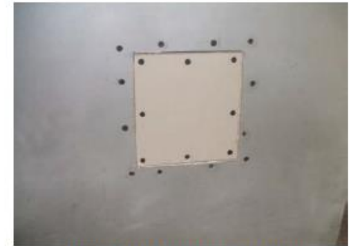
Figure 4: Apply Gypsum Panel Patch
