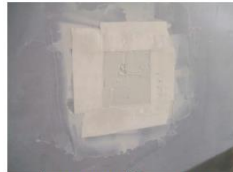
Figure 5: Tape and Finish Patched Area
