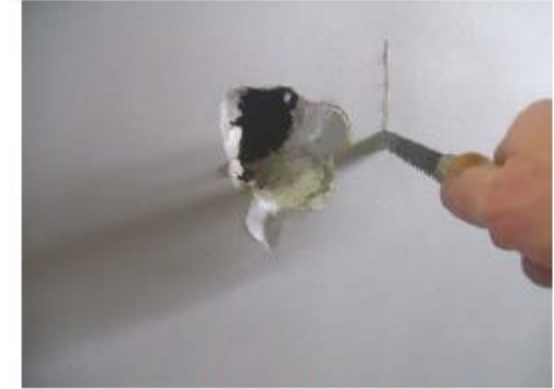
Figure 2: Square Off Damaged Area
