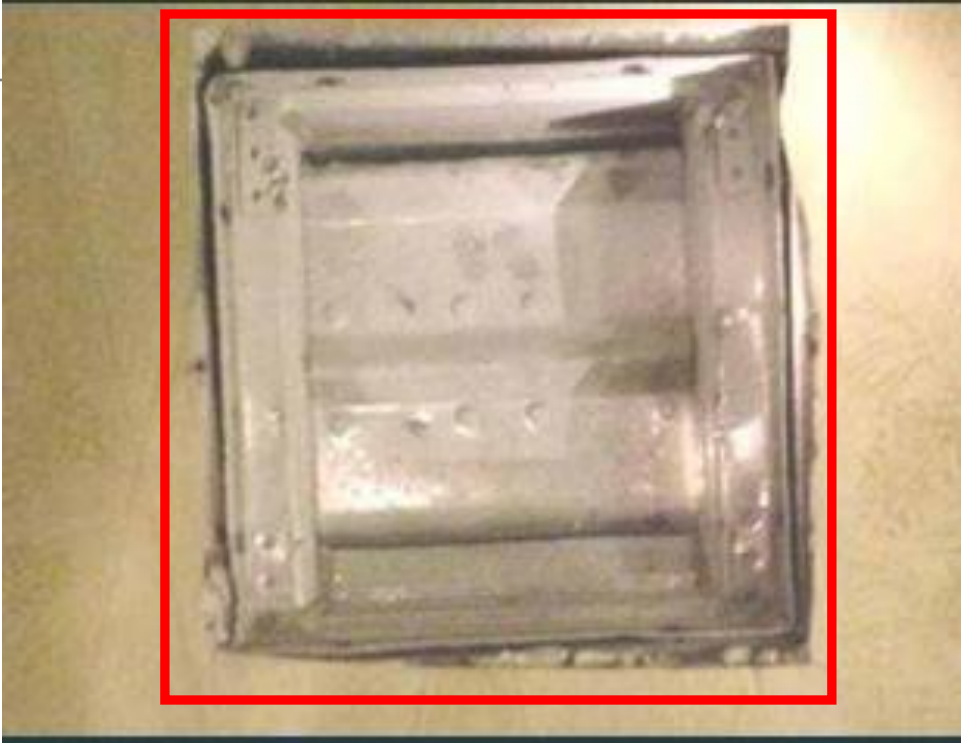
The damper not installed square, plumb, straight, it is installed racked
