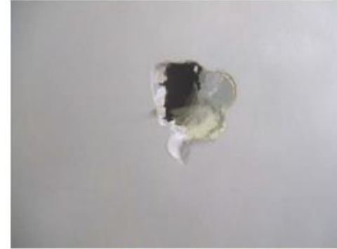
Figure 1: Damaged Gypsum Panel
