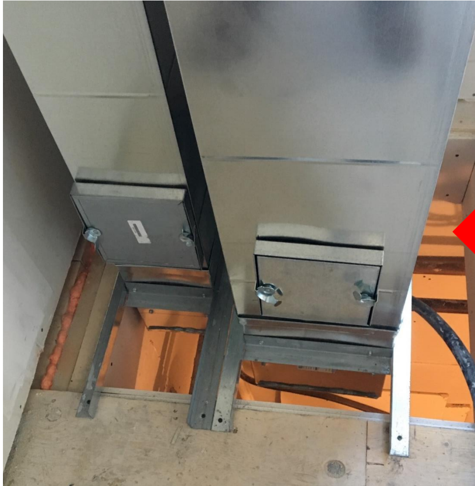
Fire Damper Annular Space?
