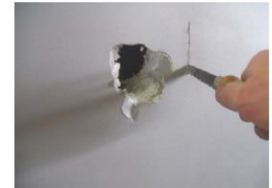
Figure 2: Square Off Damaged Area
