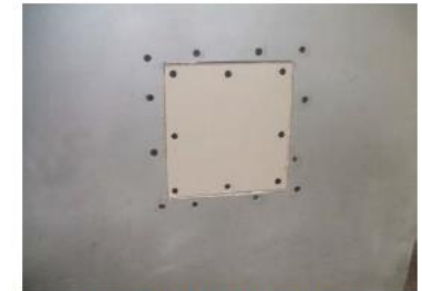
Figure 4: Apply Gypsum Panel Patch
