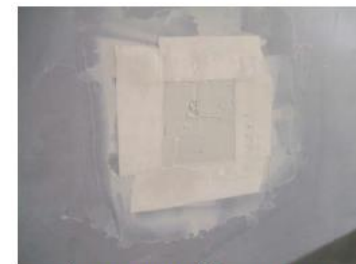
Figure 5: Tape and Finish Patched Area
