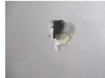
Figure 1: Damaged Gypsum Panel
