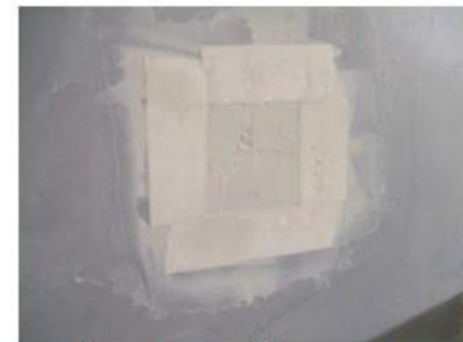
Figure 5: Tape and Finish Patched Area
