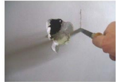
Figure 2: Square Off Damaged Area
