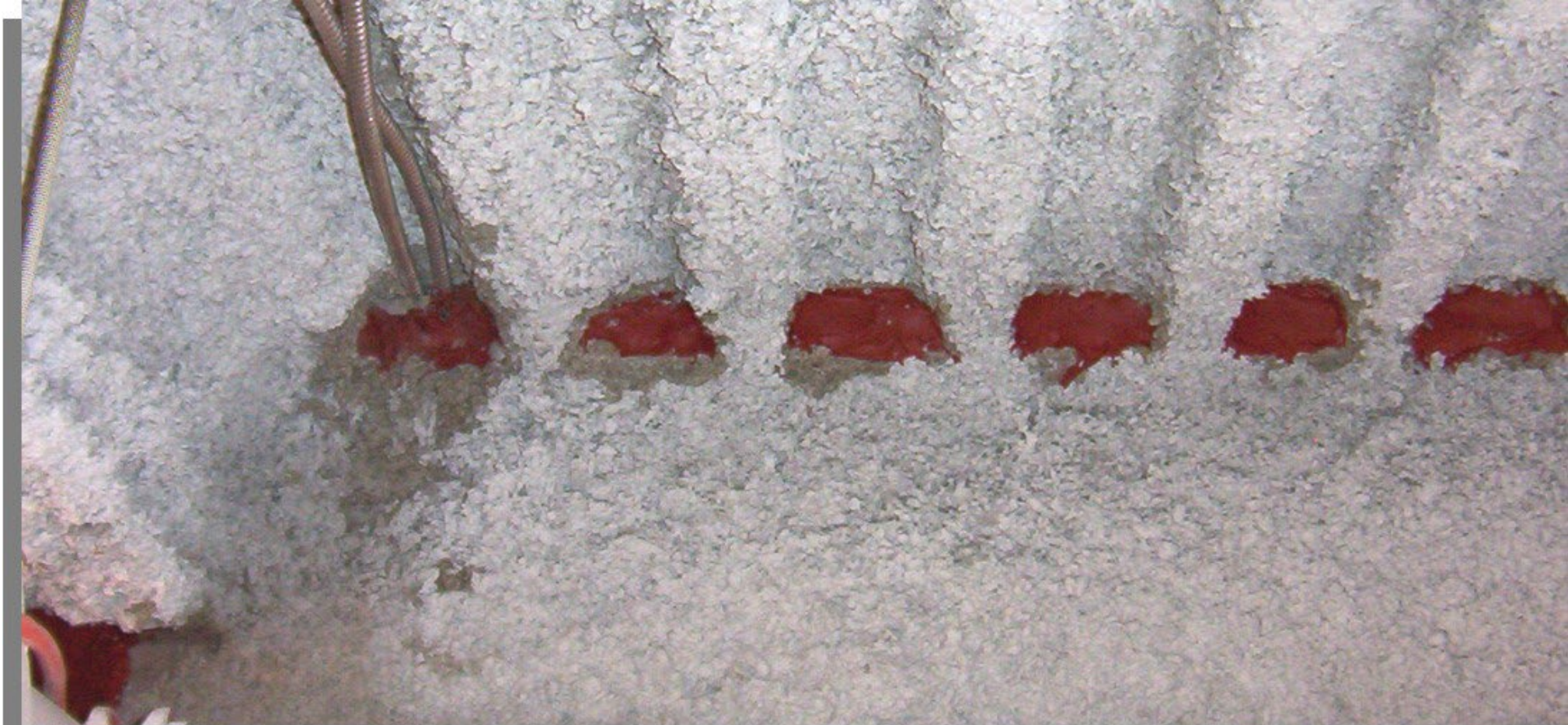
Firestop Solutions Photo
