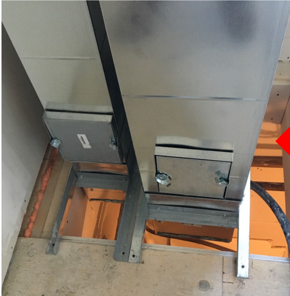
Fire Damper Annular Space?
