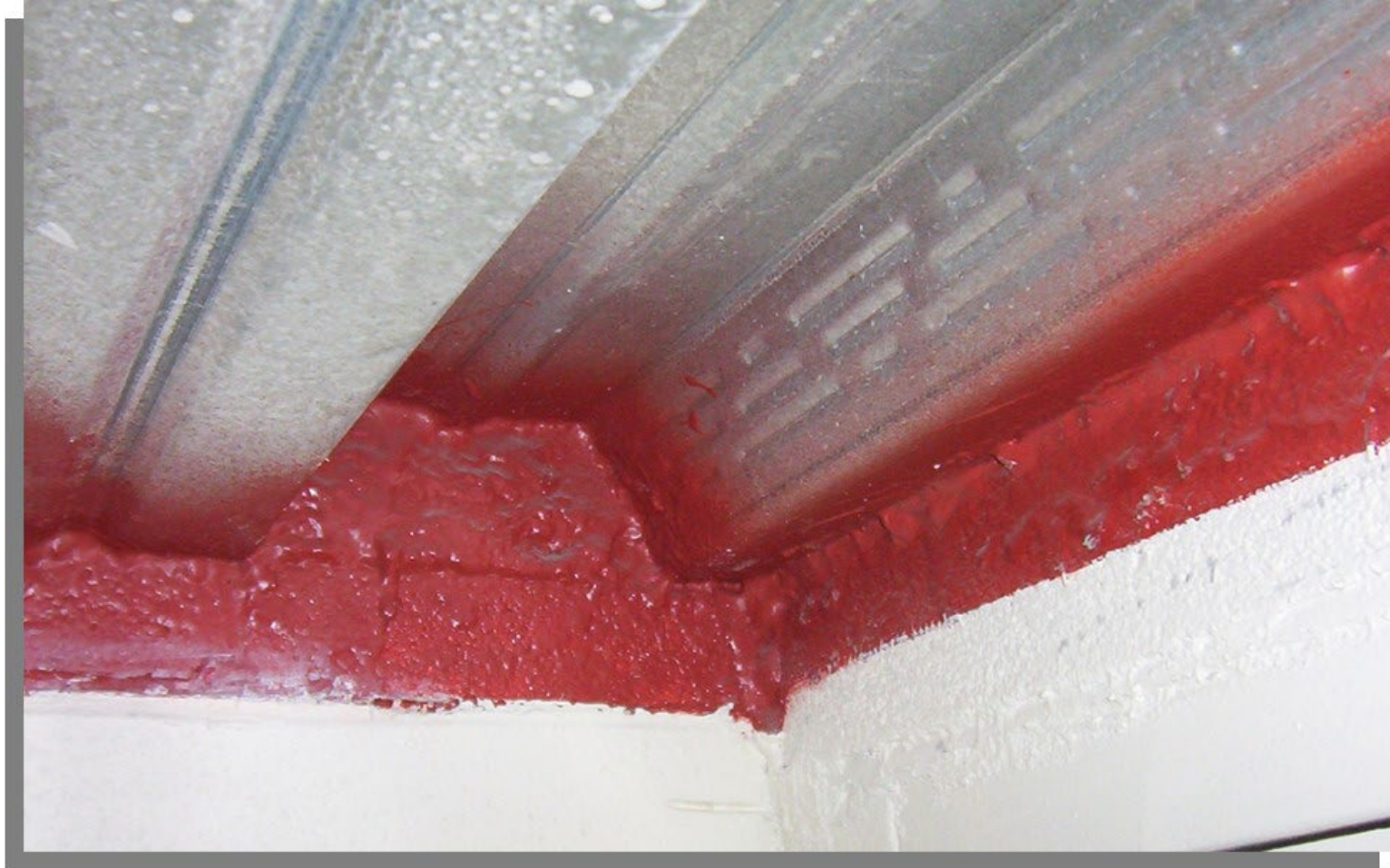
Firestop Solutions Photo
