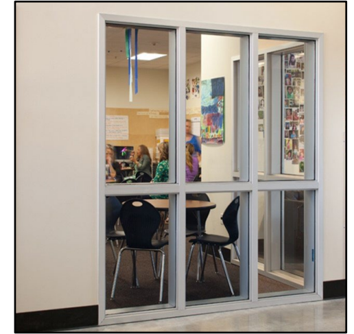
Interior Fire Windows
