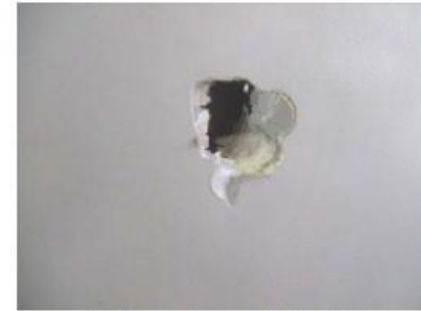
Figure 1: Damaged Gypsum Panel
