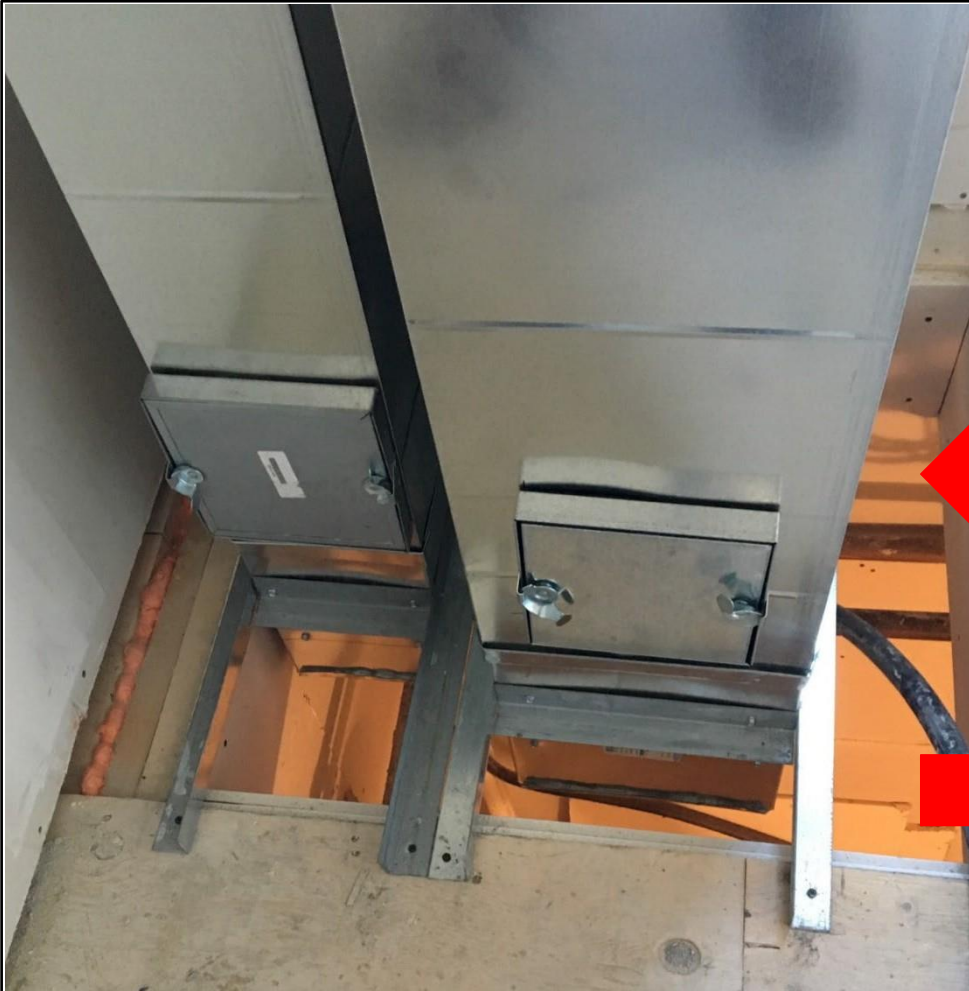
Fire Damper Annular Space?
